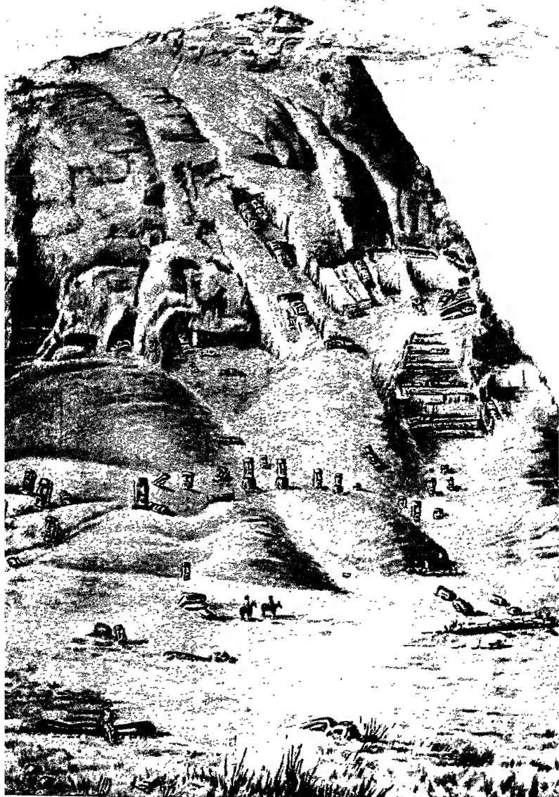
EXTERIOR OF RANO RARAKU. EASTERN PORTION OF SOUTHERN ASPECT.
